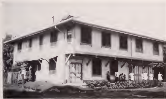
Home of Dr. and Mrs. Laubach in Dansalan. Lower floor used for mission library
